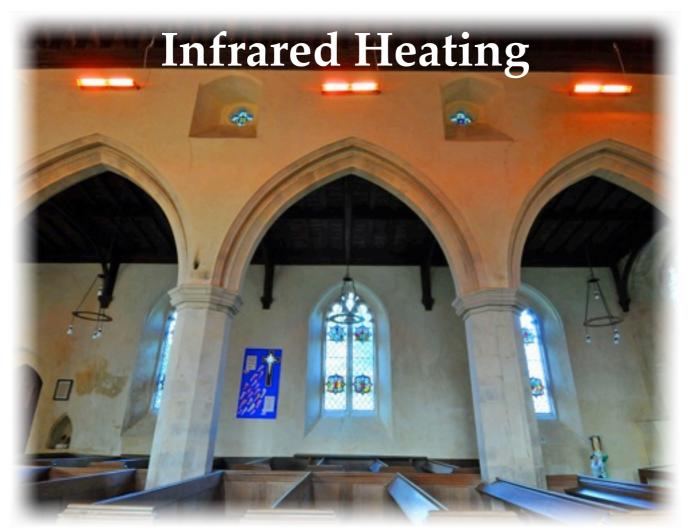
Because hot air rises, conventionally heated tall buildings will lose most of their heat up in the ceiling where it's of little use to the occupants. EHS radiant heaters counter this problem. They work by heating objects rather than the air, so people quickly become warm without wasting energy.
